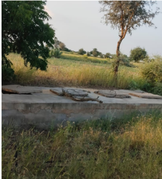
Rainwater harvesting structure at Mokheri
