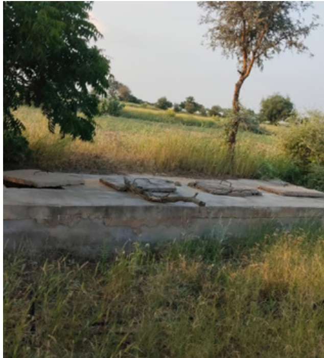
Rainwater harvesting structure at Mokheri
