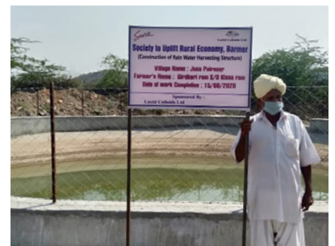
A pond with a capacity of 405 cubic meters has been constructed in Juna Patrasar Village
